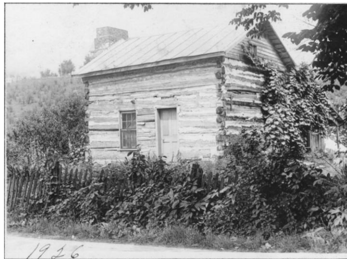
Vintage view of the Miller-Leuser Log House, dated 1926. Notice open hillside to the west of the house, the metal roof and the open porch at the back of the house. The porch was enclosed in about 1930. ATHS Collections.
