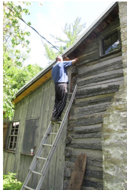
Lou Trent, chair of the Property Committee, arranged for Desmond O'Donnell to repair the chinking of the Log House.
