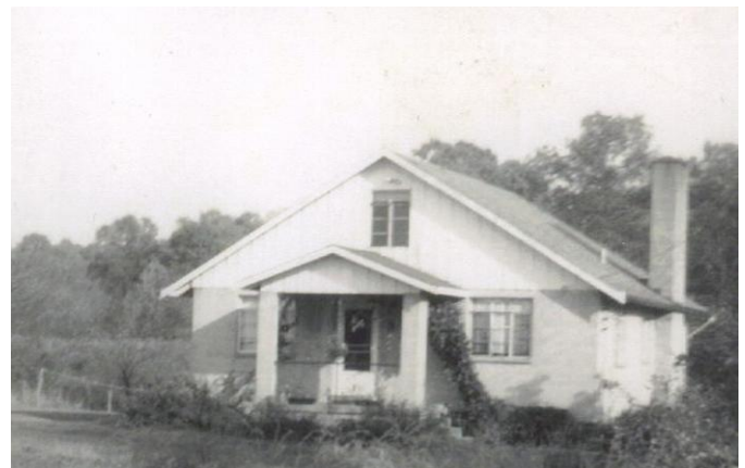
Hornschemeier house, built in 1949. Photo from the 1950s.
