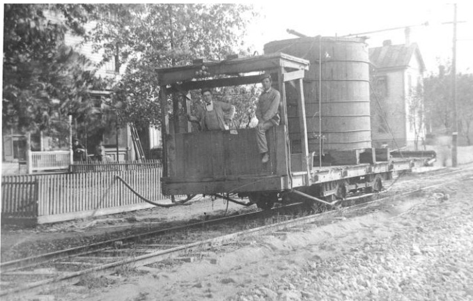
About 1910. Photo was taken along the IRT "Black Line" railroad tracks on Beechmont, at what is now the corner with Wolfangel.
